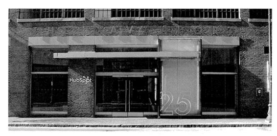
1/2" thick individual dimensional letters & graphic element, Logo pinned 3/4" off brick facade. Material either chrome plated fabricated brass letters or brushed stainless steel.
